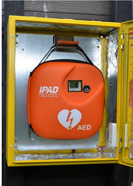
Above: Lifesaving defibrillator located in cabinet
